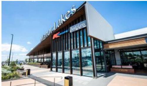
Lot 235 Taupe Street, Wyndham Vale
